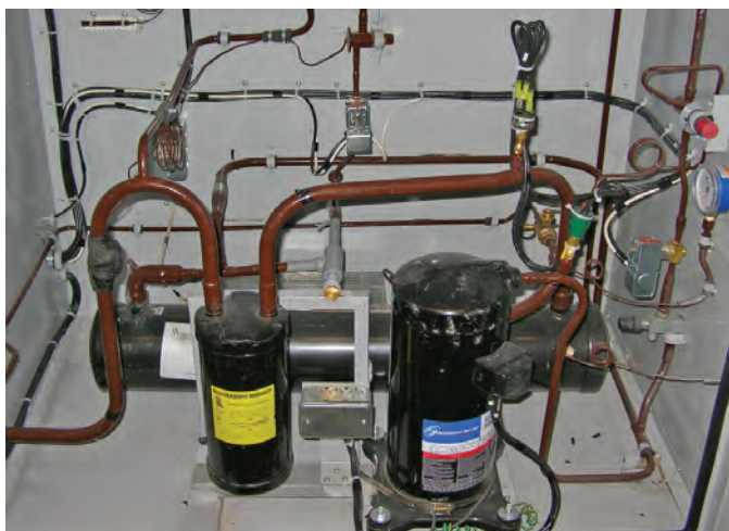
Heresite coated refrigeration piping is available for corrosion resistance.
