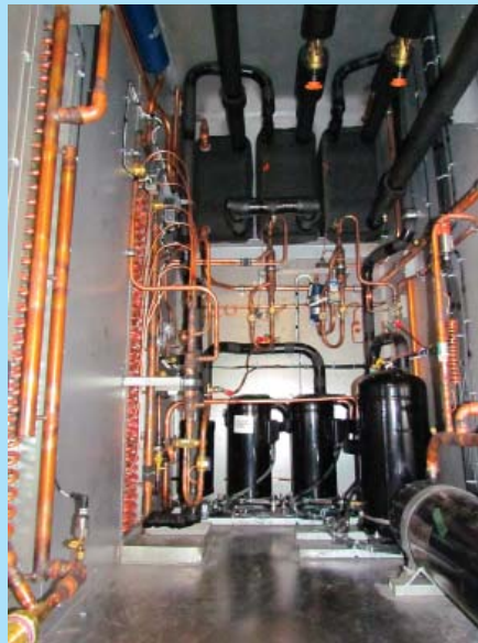
Compressor Service Vestibule
