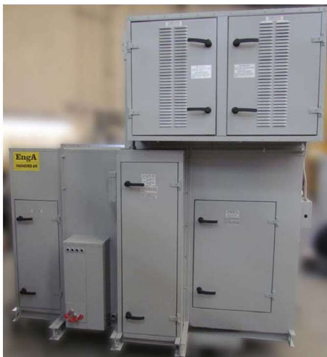
DJX100 in the vertical arrangement. This unit disassembles into five pieces to fit through a 34" wide door.
